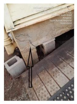
Cracked slab-note concrete block support.
