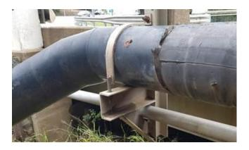
Figure D: Telecommunications conduit installed through a water pipeline bracket.
