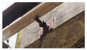
Figure E: Telecommunication conduit resting on a transverse stressing bar, increasing oxidization of the bar, and preventing the road authority from undertaking maintenance (replacement of the bar). This bar is critical to bridge integrity and safety.
