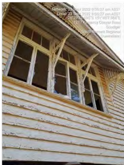
Typical damaged windows
