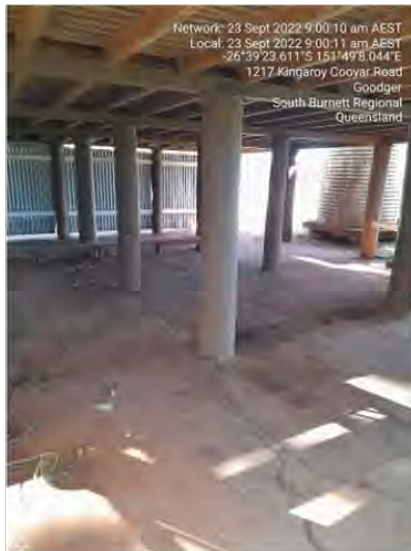
Typical timber stumps.
