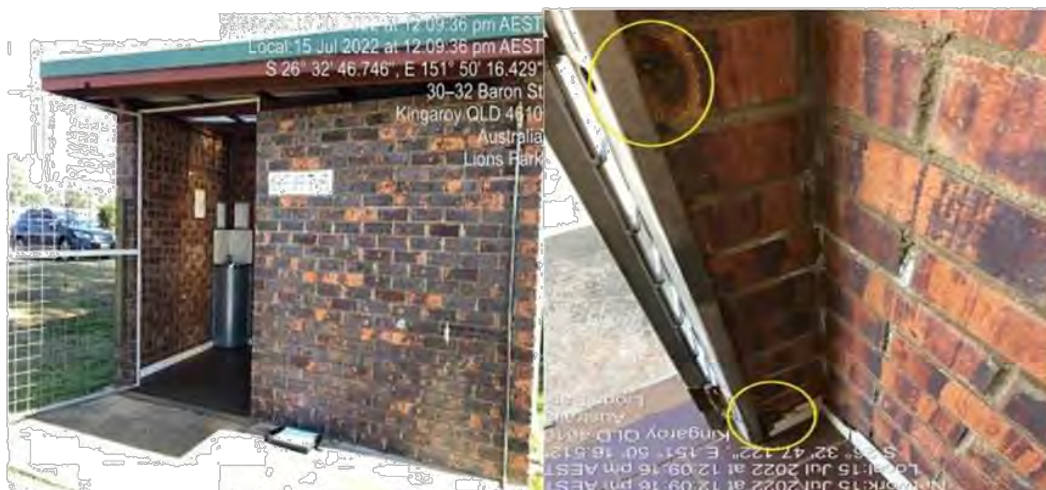
Gates swing out and cannot be secured
