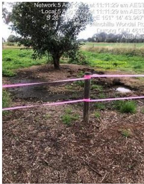
Failed trenches with ponding effluent.
