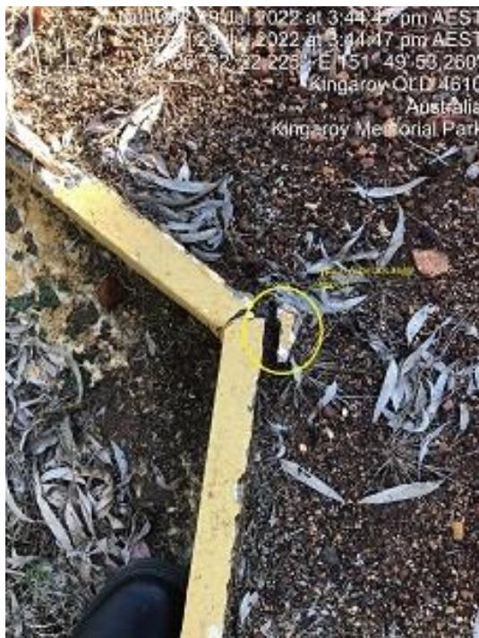
Typical damaged asbestos angle support.
