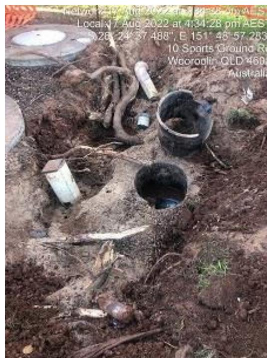
Tree roots and damaged pipework.
