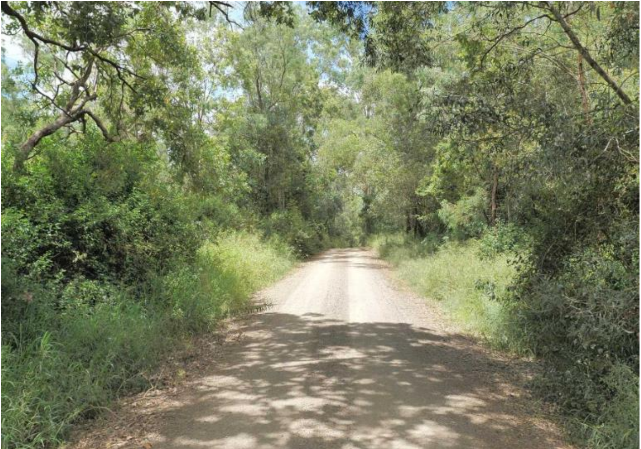
Figure 1 – Tim Dwyer Road, South Nanango – CH0.06km – example of 5C Access Track section with gravel placed.
