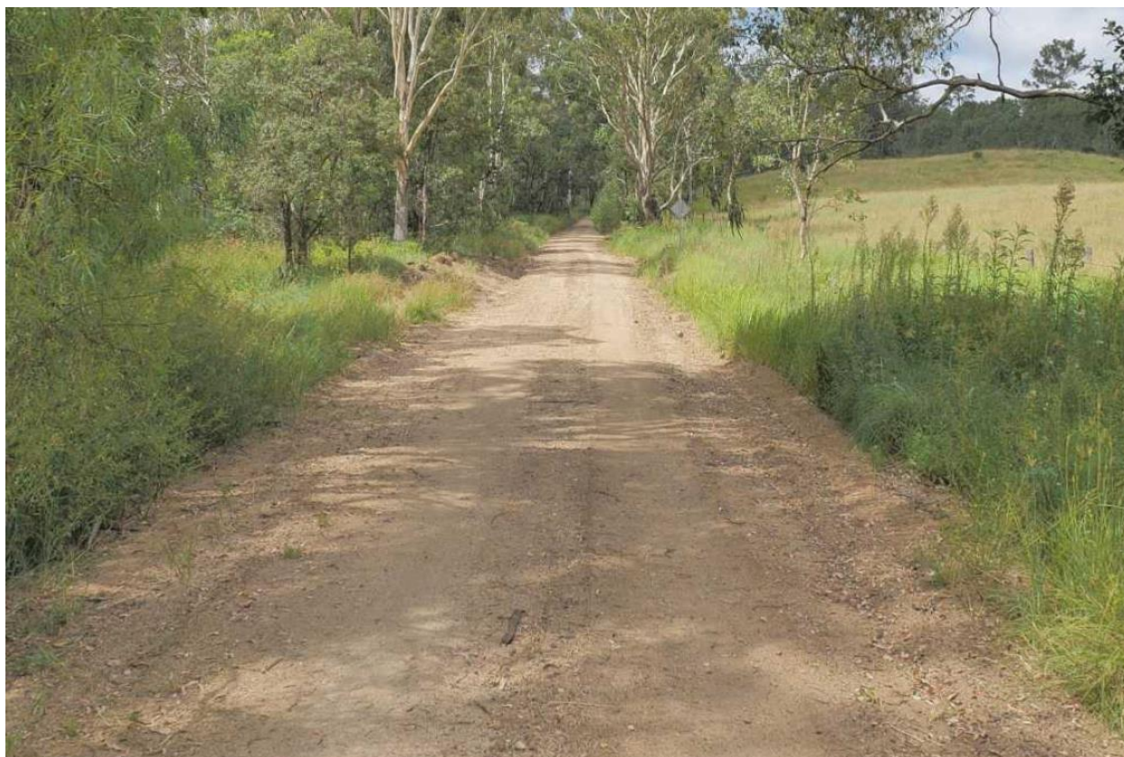
Figure 1 Tim Shea Creek Road – CH0.7km – example of 5C Access Track section with gravel placed
