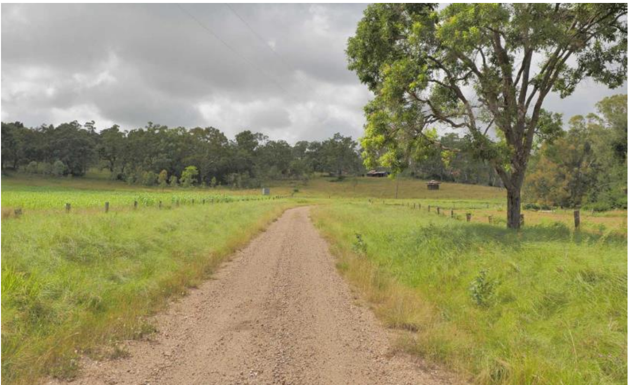
Figure 1 – Wengen Creek Road, Wengenville – CH0.4km – example of 5C Access Track section with gravel placed.
