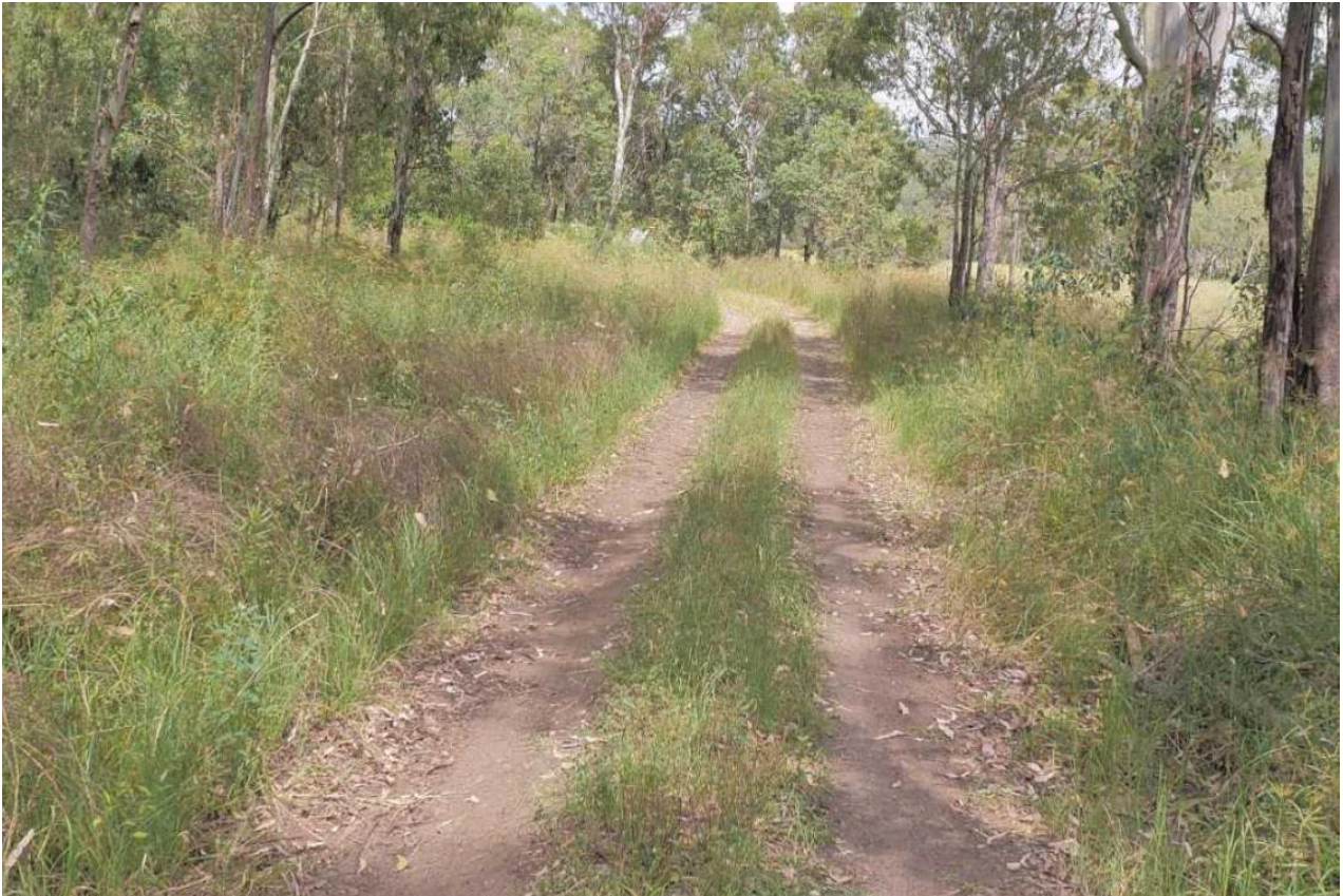
Figure 2 Tim Shea Creek Road – CH4.0km – example of 5C Access Track section – No gravel placed.
