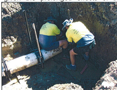
Repairing the Raw Water Intake
