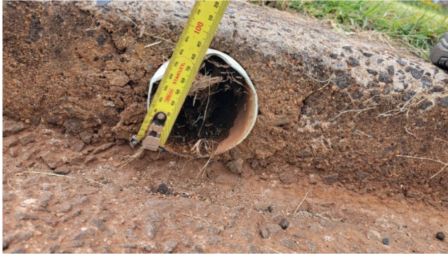
Figure 11: Pre-Development Kerb and Channel Discharge Point.
