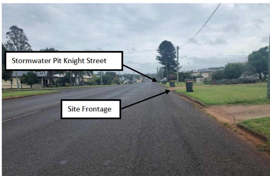
Figure 4 – Site Photo of Kingaroy Street Kerb and Channel.
