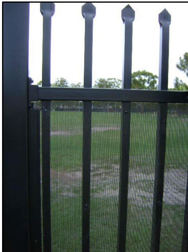
Picture 6.2: Mesh infill panel fixing on a Type 1 Security Fence
