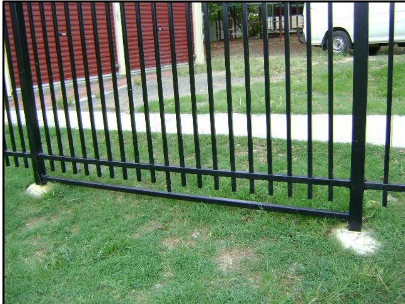
Picture 6.3: Type 1 Security Fencing with infill bar
