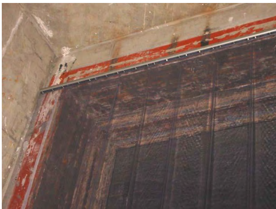
Picture 3: Mounting of 500 Series Acoustic Track.
