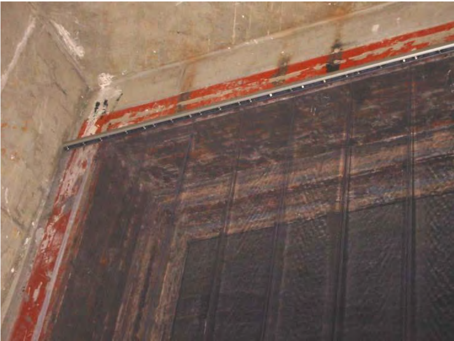
Picture 3: Mounting of 500 Series Acoustic Track.
