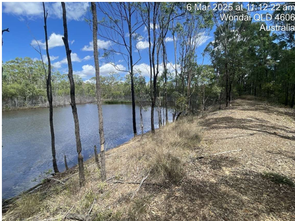
Figure 7 – Site Photo – On-site Retention Basin.
