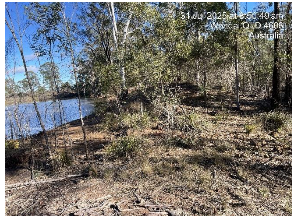
Photo 6. Eastern side of retention basin
