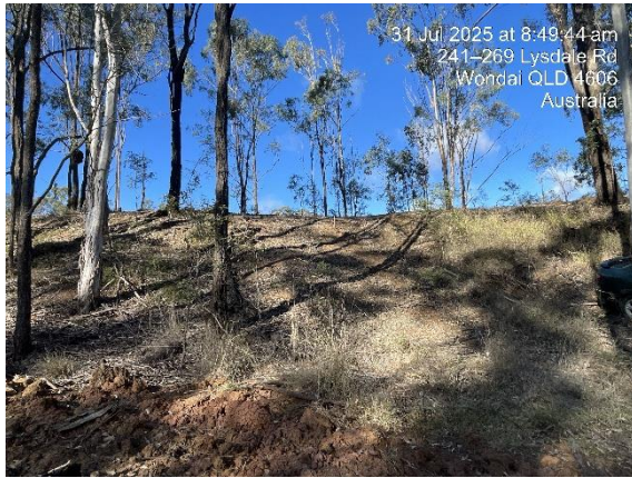
Photo 5. Existing earth bund south of the retention basin
