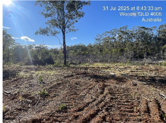
Photo 2. Development site – partial clearing of trees
