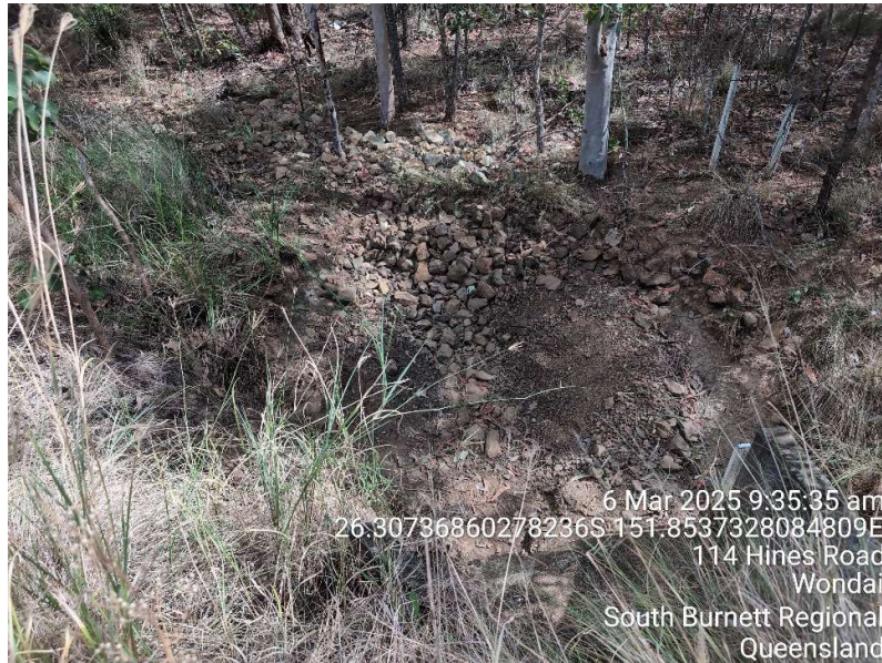
Figure 13: Concrete culvert outlet – from above (Cnr Hustons & Hines Road).
