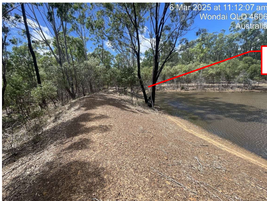
Figure 8 – Site Photo – On-site Retention Basin – Looking Towards Overflow Outlet.
