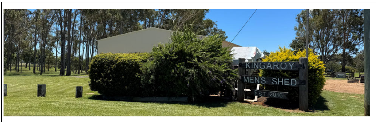
PHOTOGRAPH 5 - View of the Kingaroy Men's Shed to the south of the development site area.
