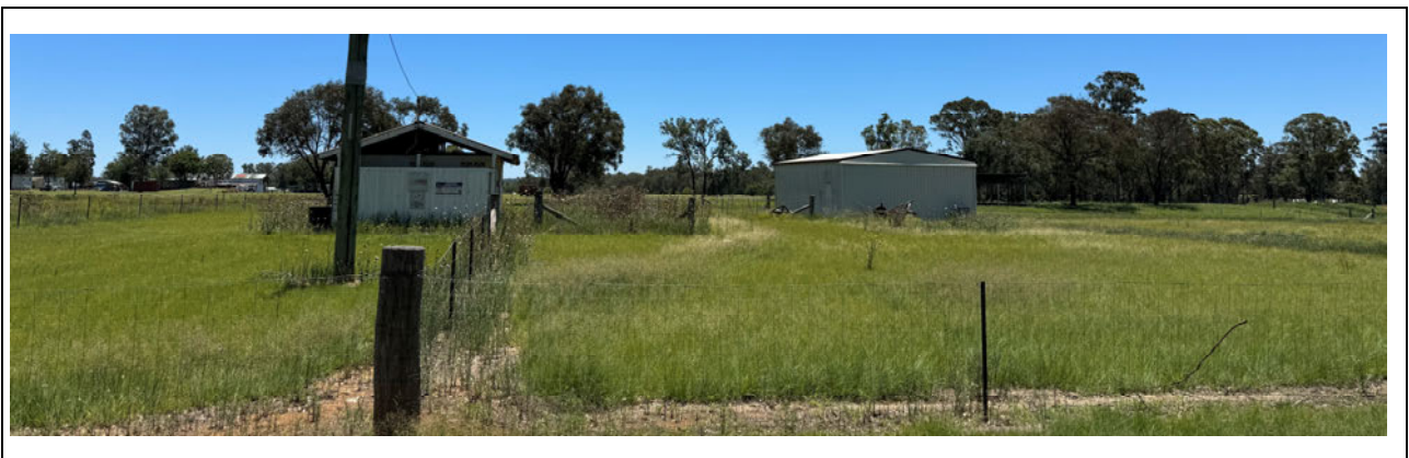
PHOTOGRAPH 4 - View of the South Burnett Junior Motorcycle Club to the east of the development site area.
