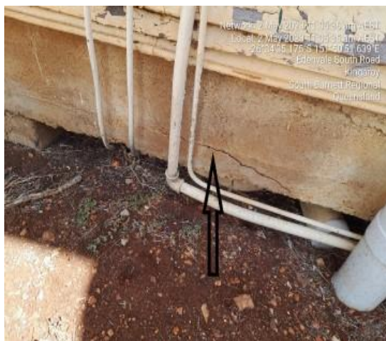
Cracked slab.
