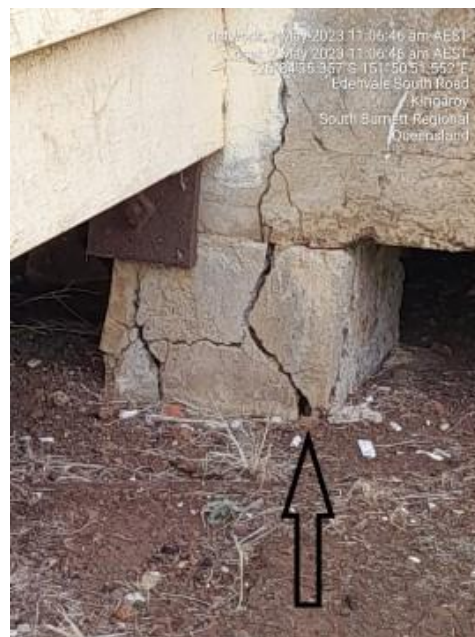
Slab/stump deterioration.
