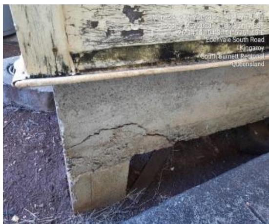
Slab damage.
