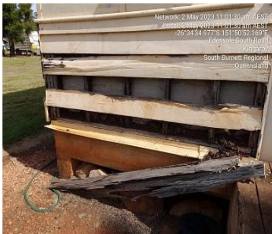
Termite damaged to weatherboards.
