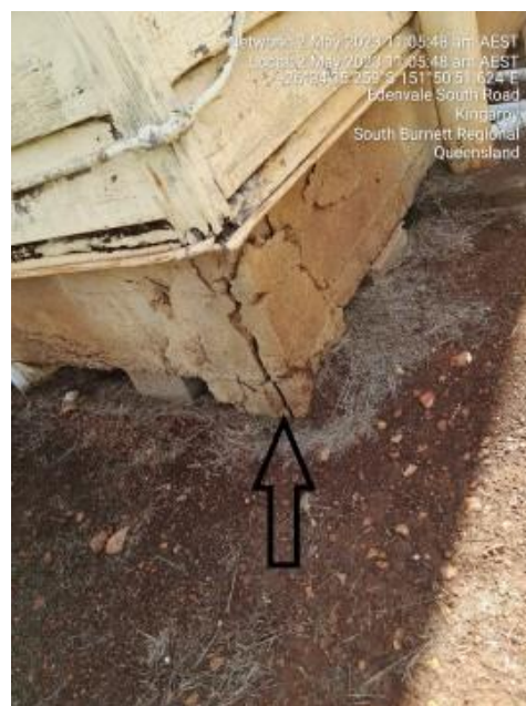
Slab damage.
