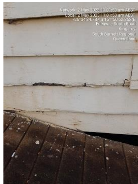
Typical rot to weatherboards.
