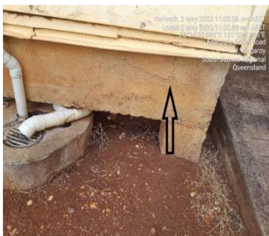
Cracked slab.
