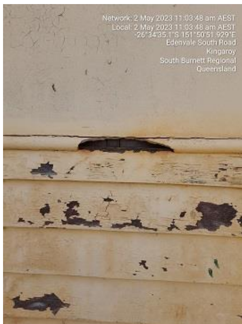
Cover strip and paint in poor condition.
