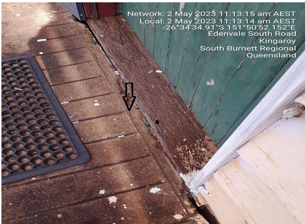
Eastern concrete access ramp has moved away from the building.
