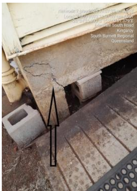
Cracked slab-note concrete block support.
