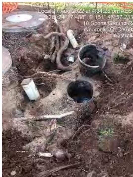
Tree roots and damaged pipework.
