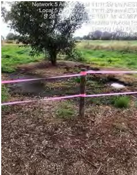
Failed trenches with ponding effluent.
